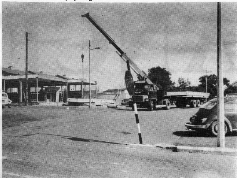
● Workers dismantling the pre-fab at Old Bawn Road.
