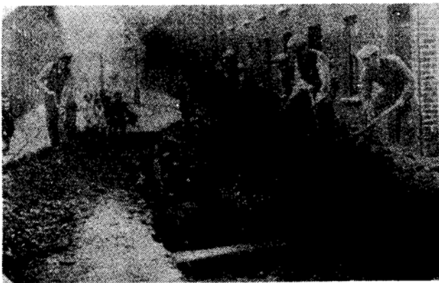
Outdoor relief workers laying drains.
