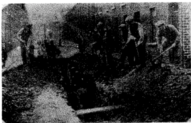
Outdoor relief workers laying drains.
