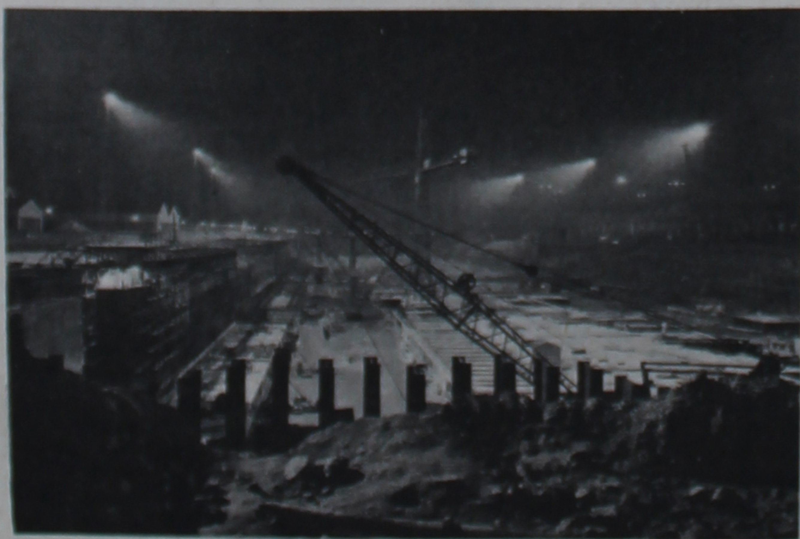
Building a new dock by night
