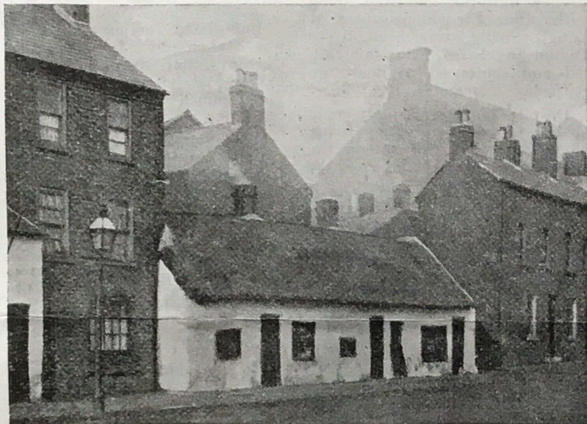
The old cottage in Frederick Street, Belfast, in which Lord Edward Fitzgerald was safely hidden between the roof and the rafters while on the run in 1798. It was demolished some years ago.
