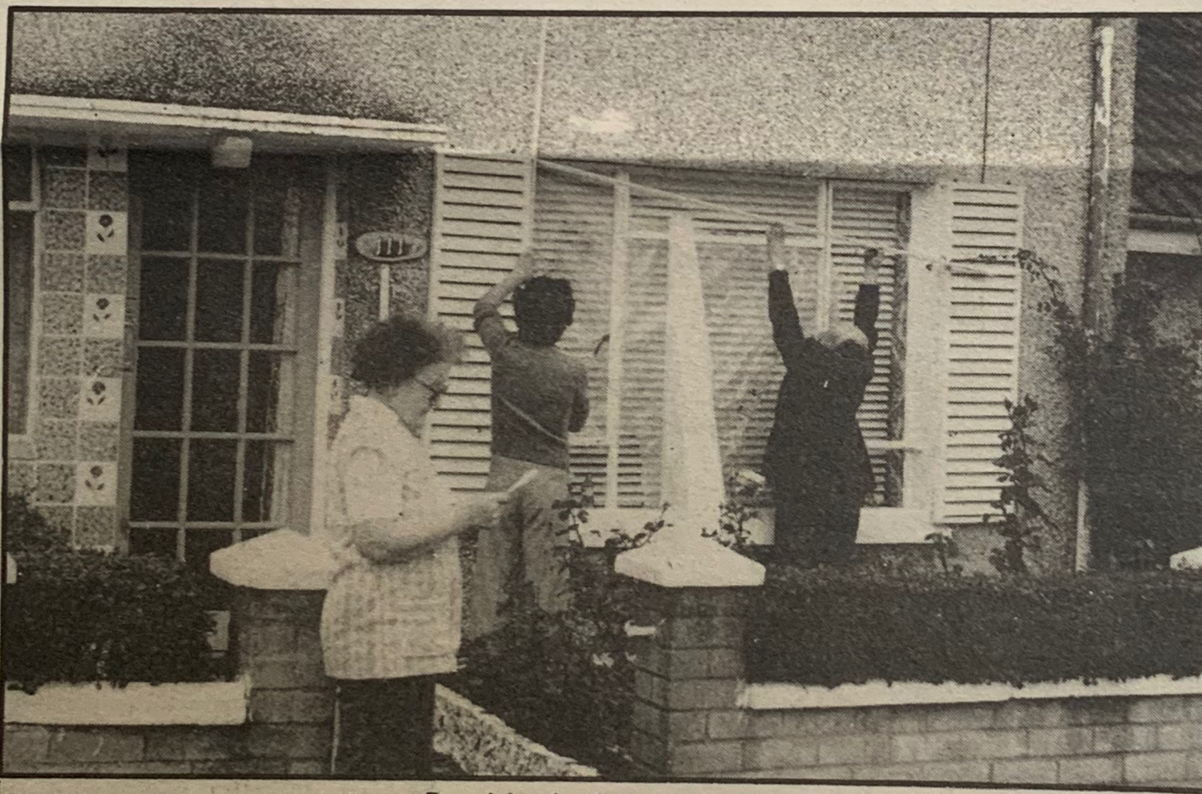
Repairing broken windows
